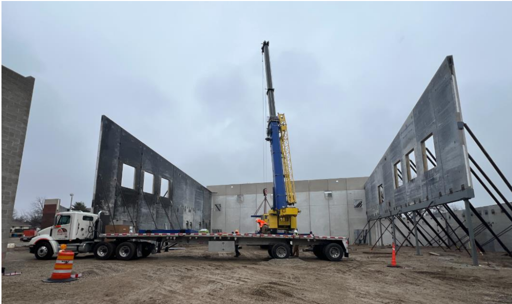
PRECAST ERECTION
